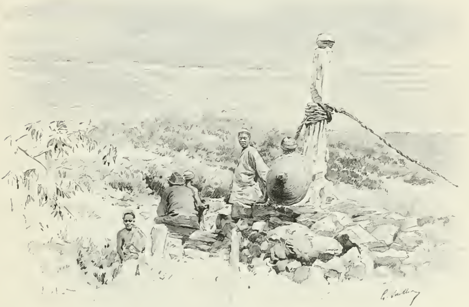
Attachment of Cord Bridge at Piao-tsen.
